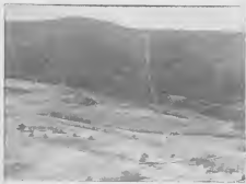
The pipeline is easy to follow when it goes over mountains through woods. When it was first laid, the trees and underbrush were cut away. However, in flat country where the pipeline is buried, the job is harder.
